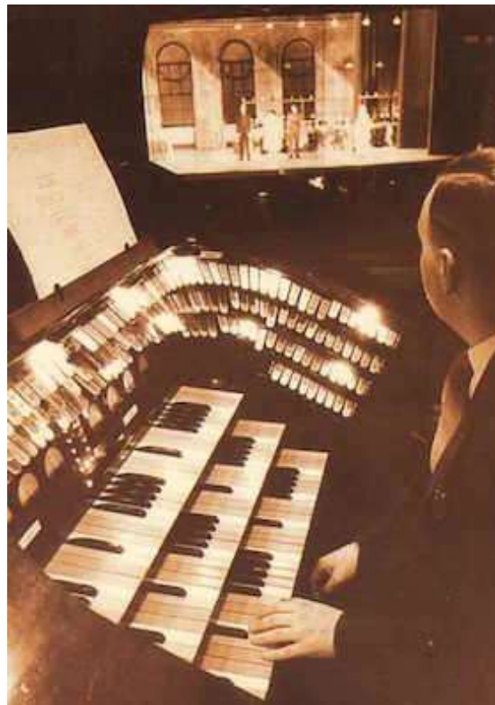
An operator at the controls of a remote Strand Light Console with full view of the stage-action. The 17 note key octaves and 5-1 black note configurations would befuddle the best of organists.
