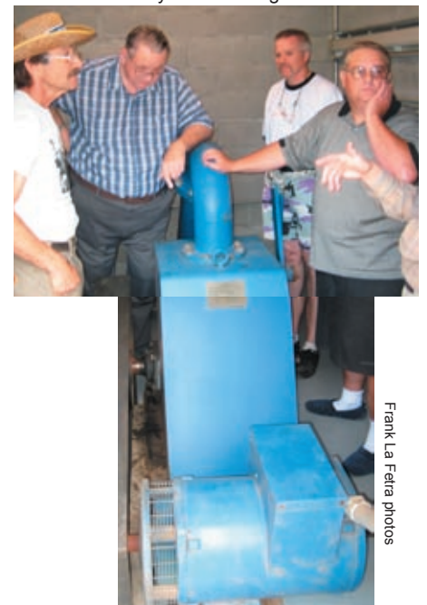
Stream that feeds Power Plant 90-feet below & 12 KW Hydro Electric generator
